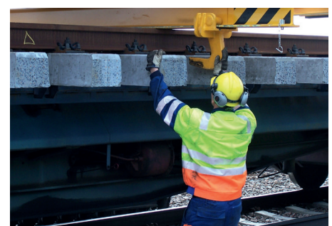
Pushing the load hooks in position from the ground
