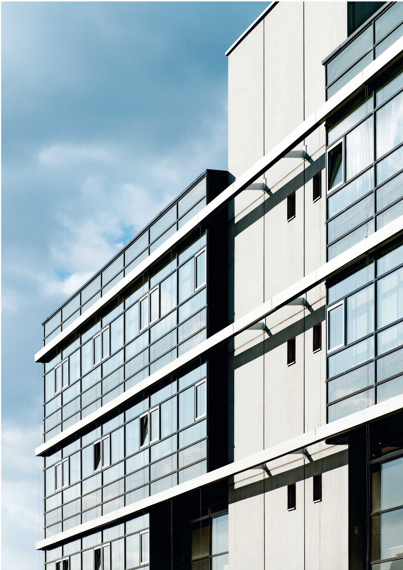
↑ Technical Development Center
