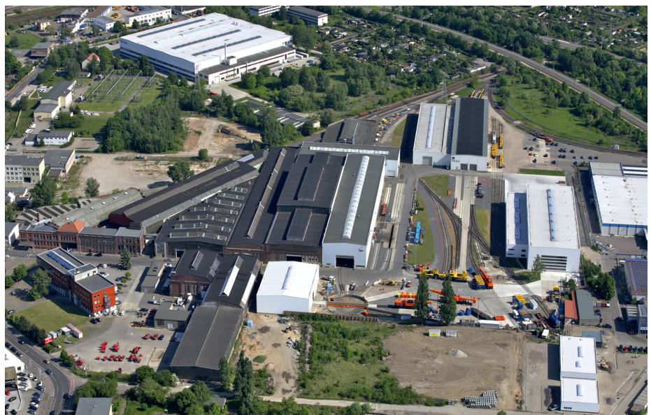
↑ Kirow production facilities in Leipzig
