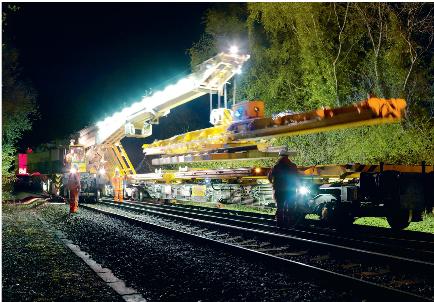
↑ Unloading a switch section from the Switch Tilter in England
