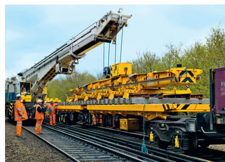
↑ Crane crossbeam is linked with the points section
