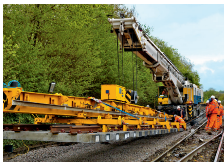
↑ Installation of the points section by the Multi Tasker
