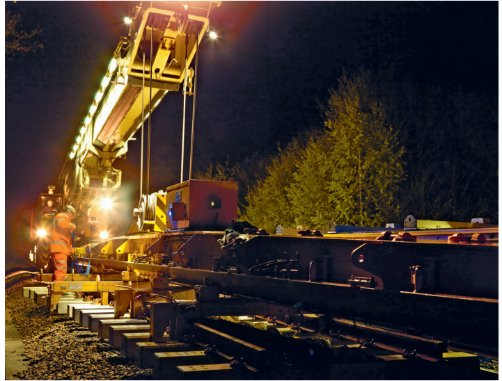
A specialised lifting beam lifts the switch section by means of the Cross Beams fixed onto the panel
