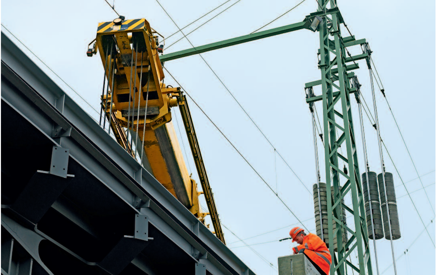
↑ Working below catenary
