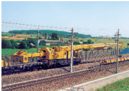
↑ Laying of track sections with restricted space conditions
