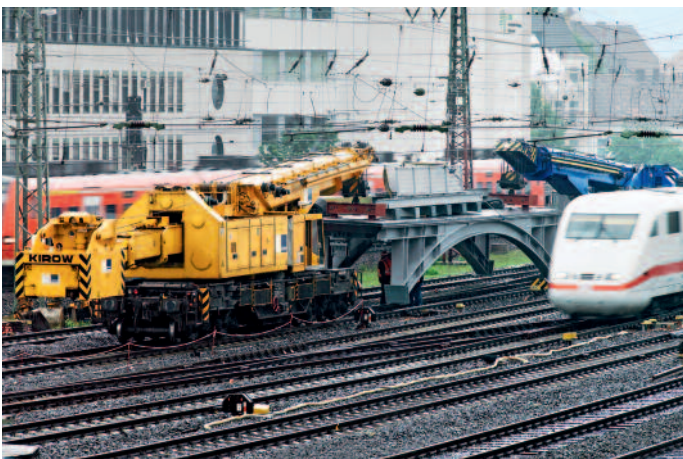
↑ Bridge construction in tandem operation
