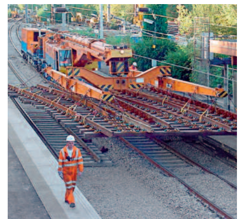
↑ Only the Multi Tasker can move such broad loads on the rail
