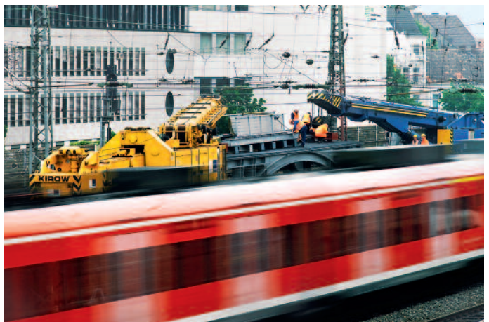
↑ No obstruction of train service
