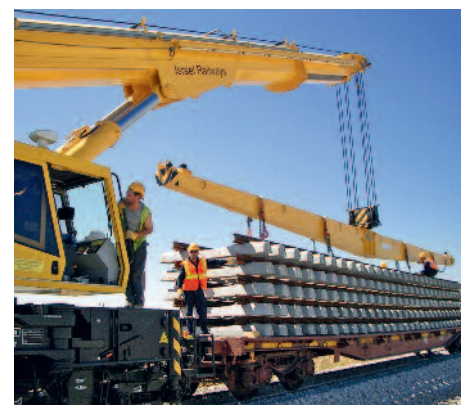
↑ The track sections are laid directly from the wagon onto the adjacent tracks
