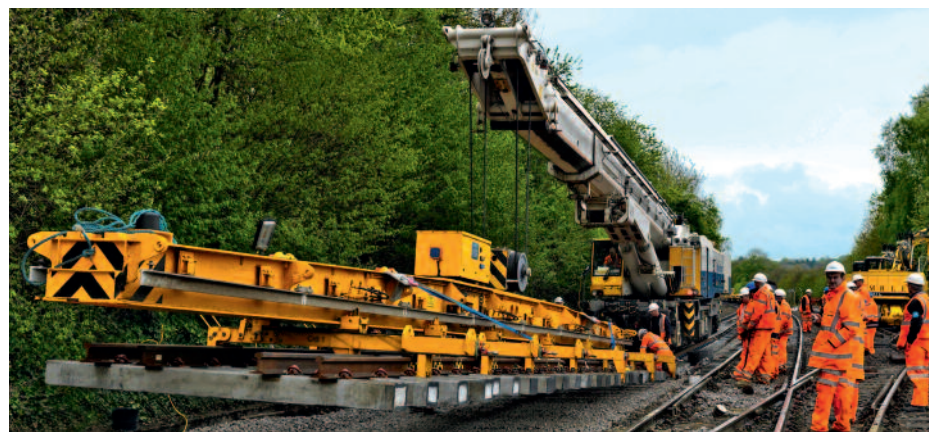
↑ Load positioning with the Self-Levelling Beam
