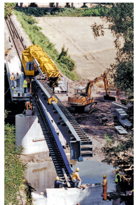
↑ Efficient erection of bridge girders
