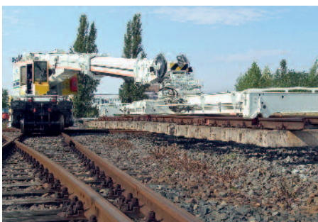
↑ Track sections can be moved by means of hydraulic beam
