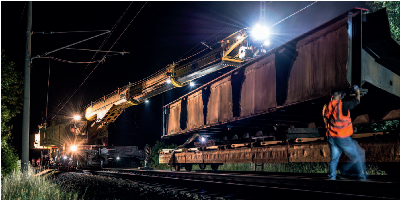
↑ Multi Tasker 1200 when lifting one of the largest auxiliary bridges of DB AG
