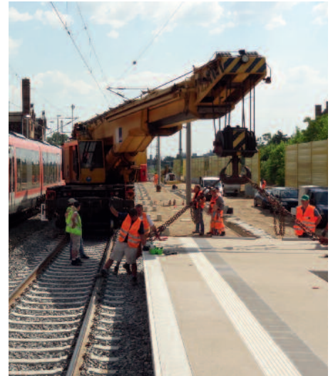
↑ Lifting concrete elements with the Multi Tasker
