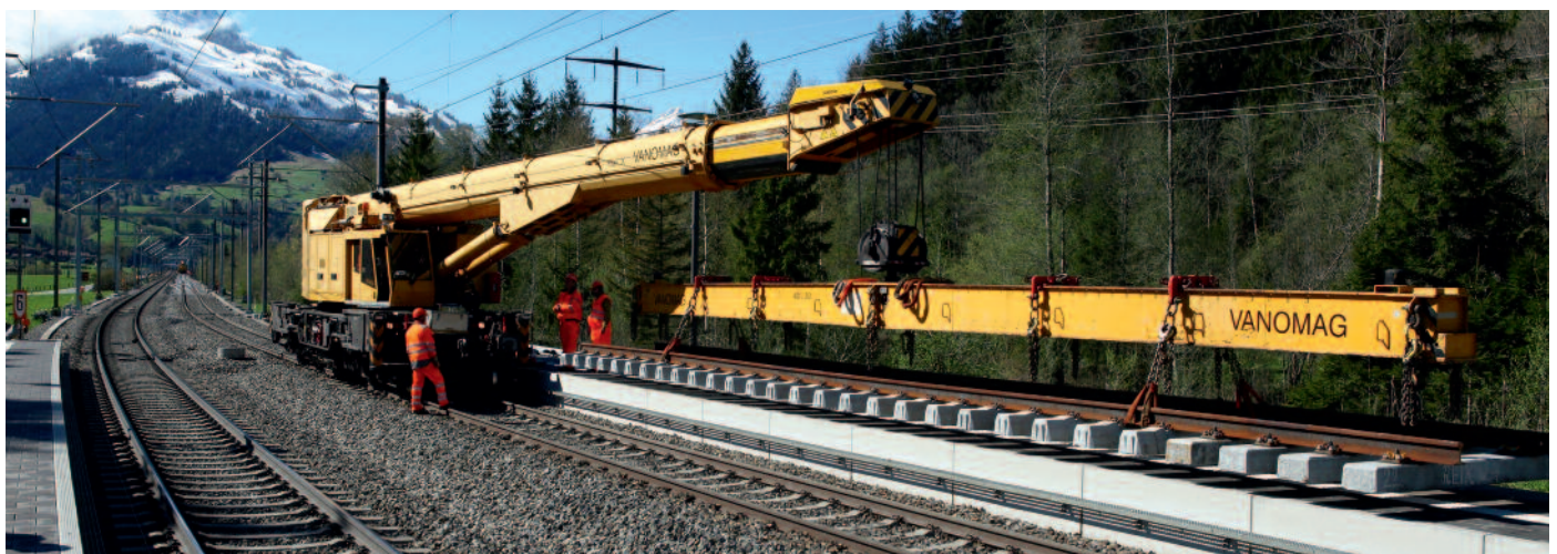
↑ Switch section lifted from the side
