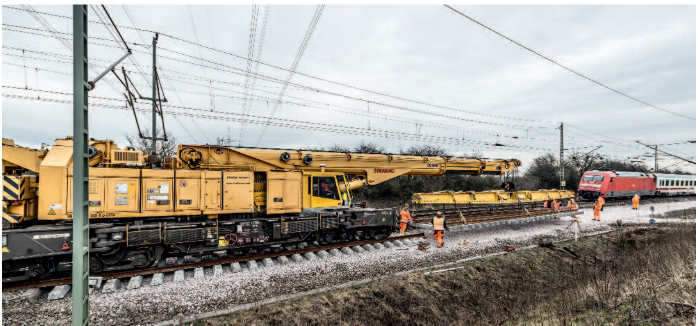
↑ Traffic continues during operations. The Multi Tasker does not affect the train traffic
