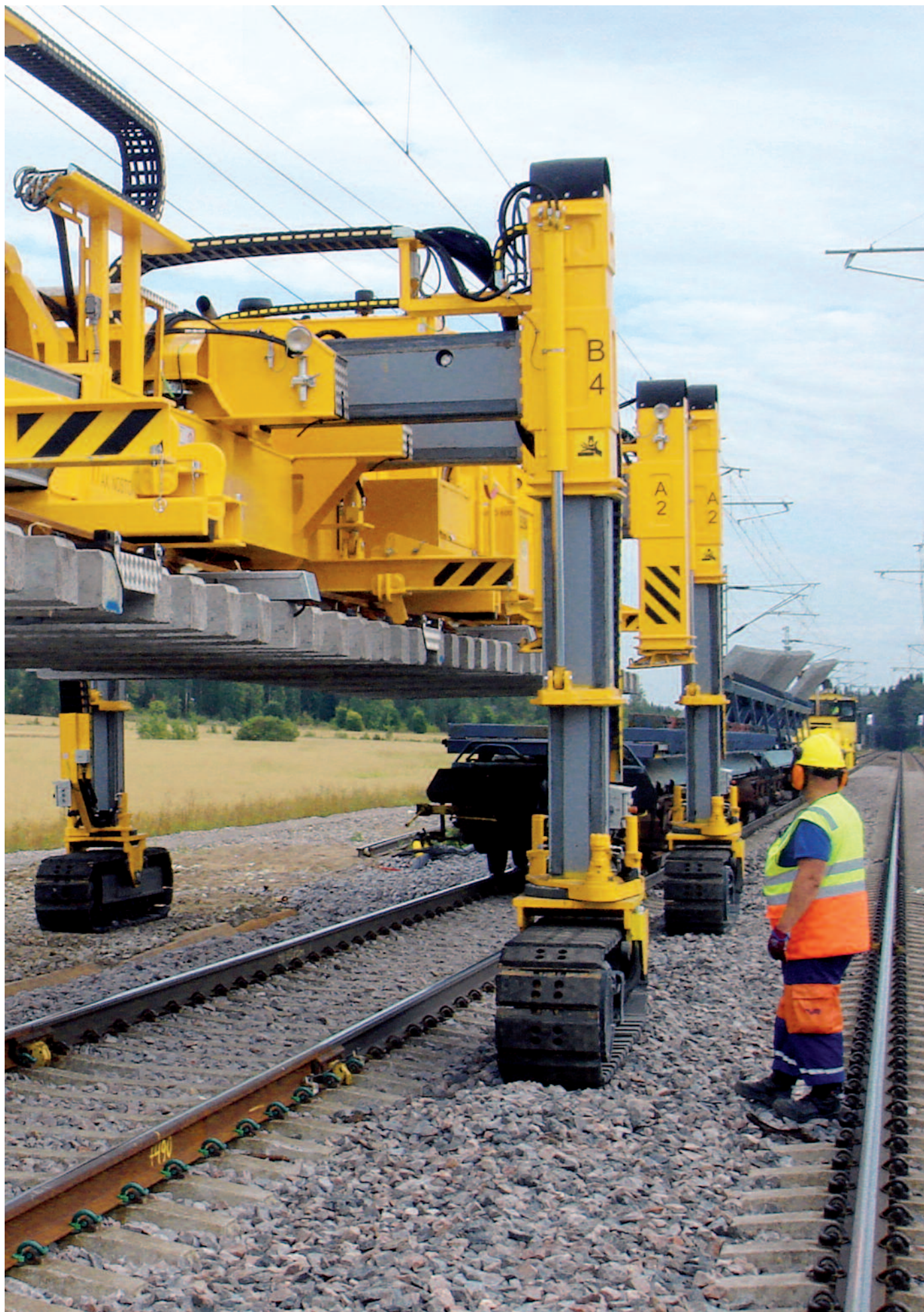
↑ Only one track is required: the DESEC Tracklayer and Switch Tilter working together
