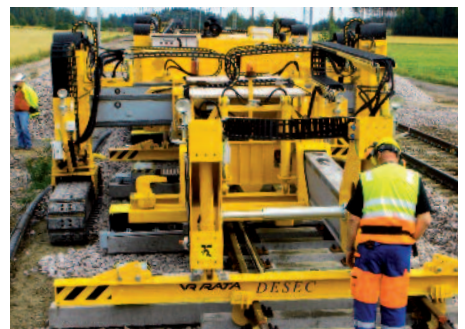
↑ Installation of panel by Tracklayer
