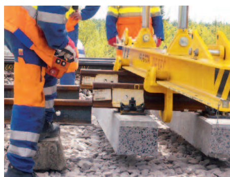
↑ The operator places the switch panel accurately standing right at the track joint
